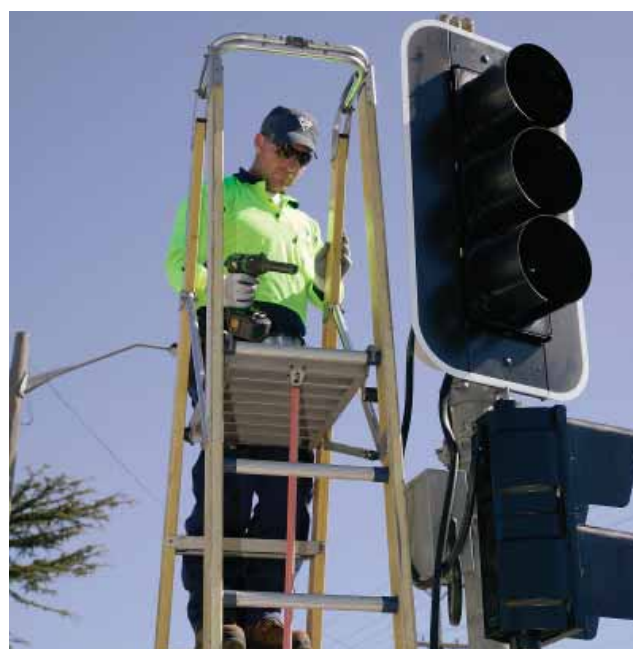
Maintenance works on traffic signals.
