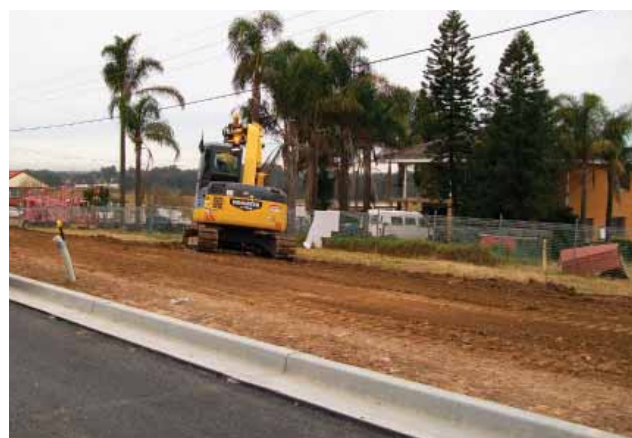
Excavators trim the verges on Camden Valley Way between Bernera Road and Cowpasture Road.
