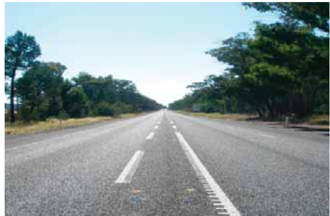
New wide centreline being trialled on the Newell Highway.
