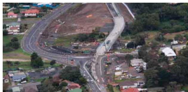
The Bulli intersection upgrade, Princes Highway.
