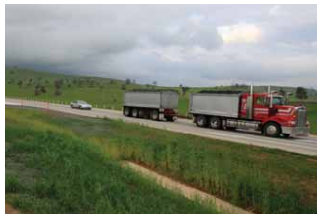
Truck on the Coolac Bypass, Hume Highway.
