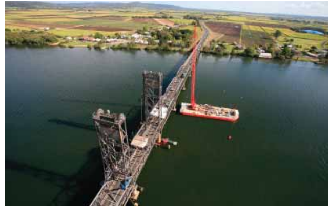
Overhaul of Harwood Bridge, over the Clarence River.
